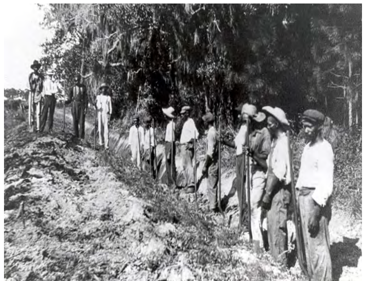
Building Roads on Sapelo Island 1920s.
