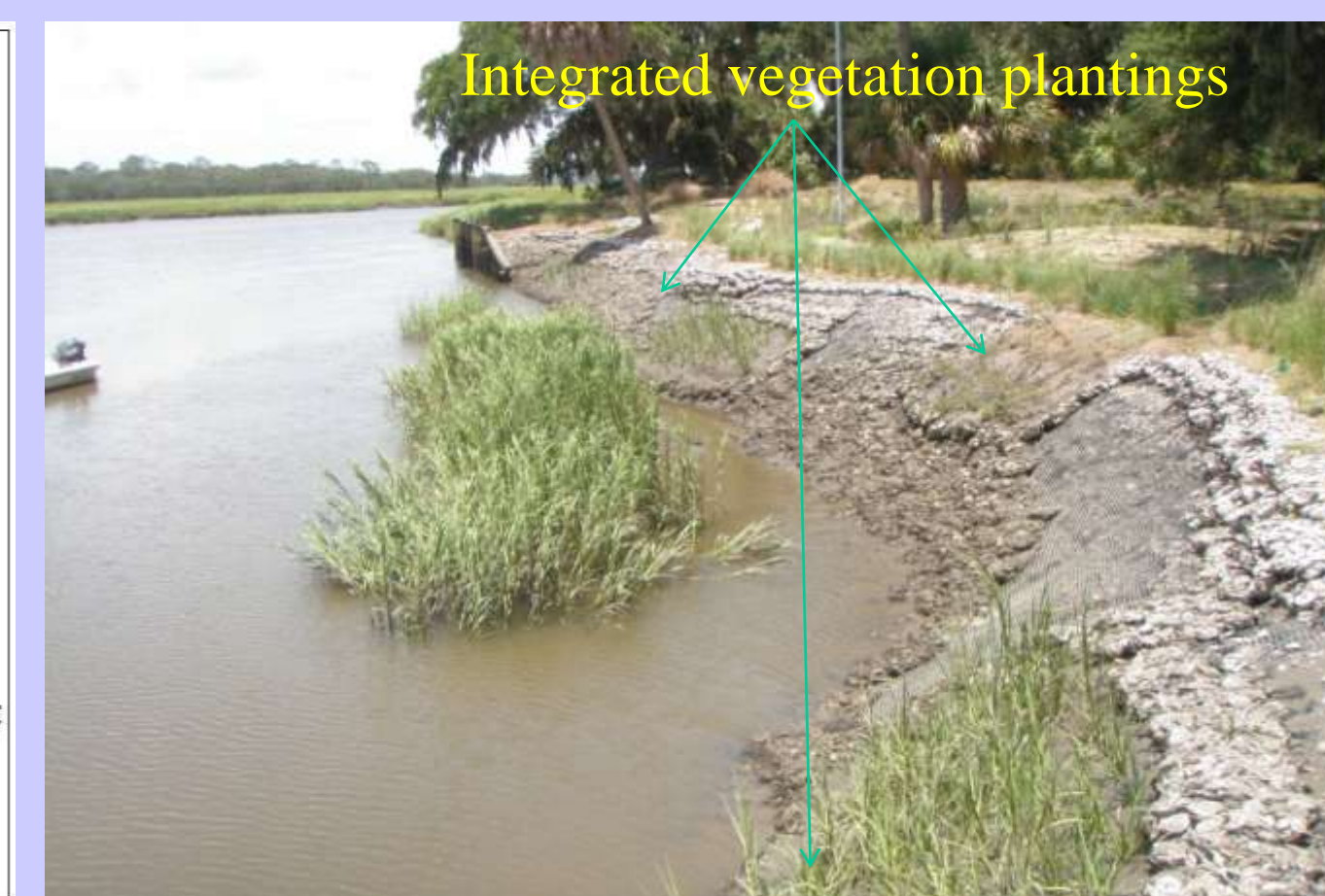
Figure 2b. Actual site (LSSI) during construction.
